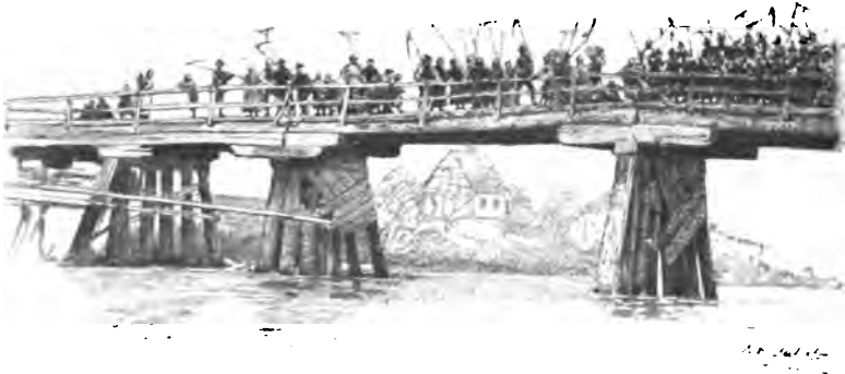
BRIDGE AT ROTTENACKER
